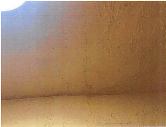
9.b Cracking
