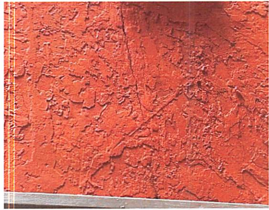
6.i Cracks in small areas
