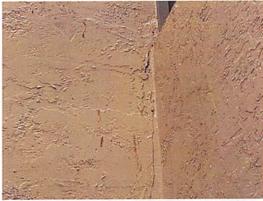
5.d Hairline cracks on walls
