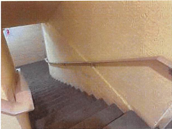
7.b.5 Guard rails in fair condition
