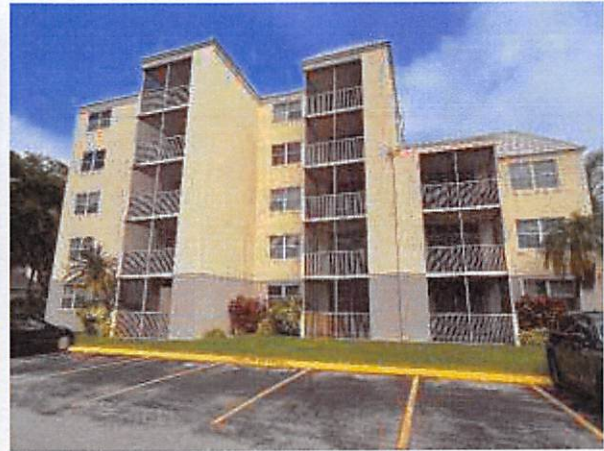
3.b Façade south side
