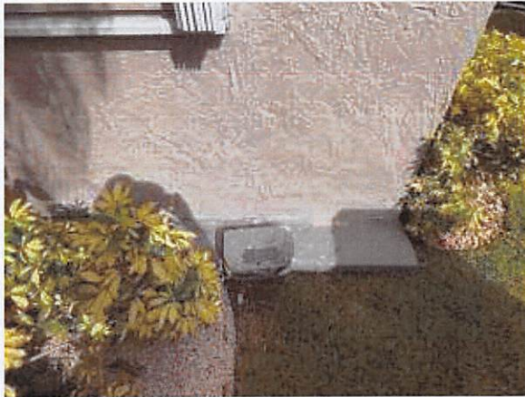
5.f Patching on walls
