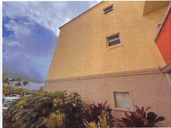
6. Masonry wall in fair condition
