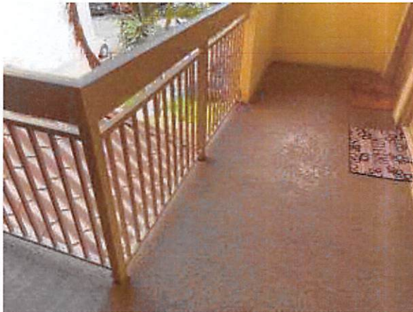
7.b.2 Balconies in fair condition
