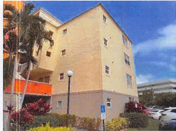
5.a Overall structure in Fair condition
