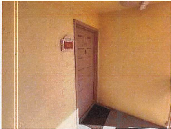
10.c Exterior doors in fair condition
