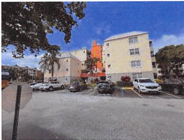
3.b Façade east side
