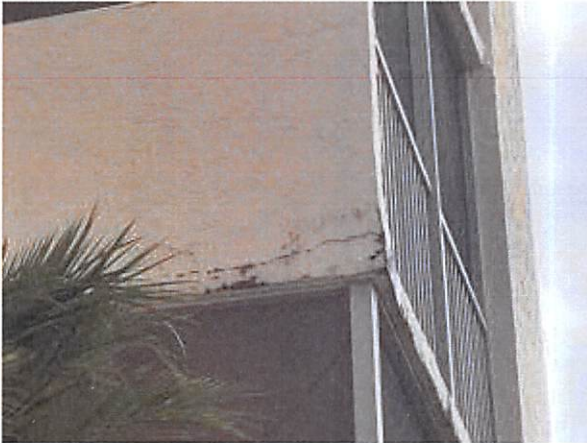
5.b Structure in fair conditions
