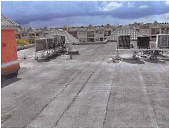
7.a.6 Roof covering in fair condition
