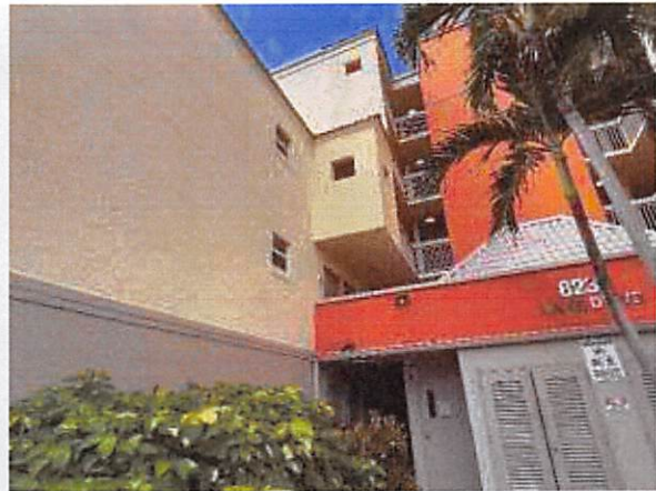
5.e Structure in fair condition
