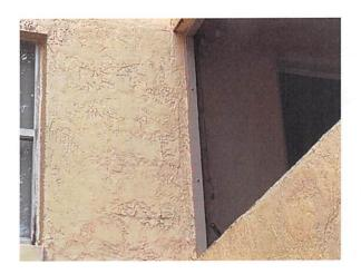
5.d Hairline cracks on walls
