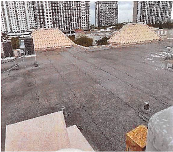
7.a.6 Roof covering in fair condition
