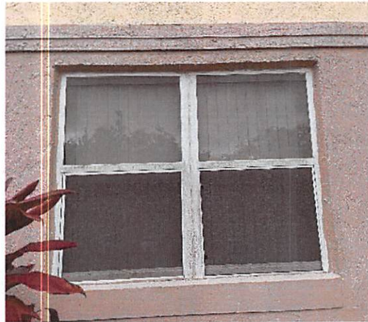
10. Windows in fair condition
