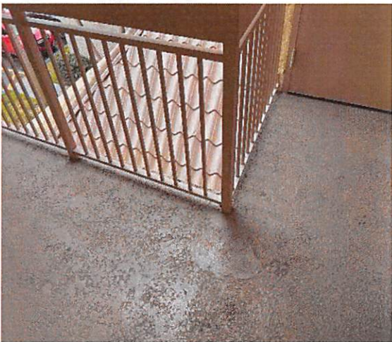
7.b.2 Balconies in fair condition
