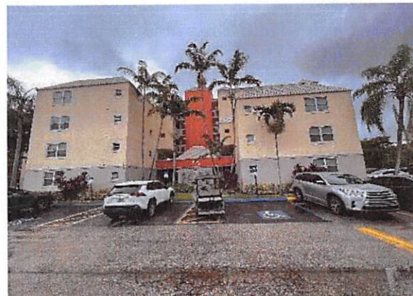
3.b Façade north side
