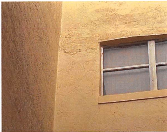
5.f patching on walls
