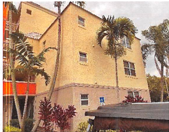
5.a Overall structure in Fair condition
