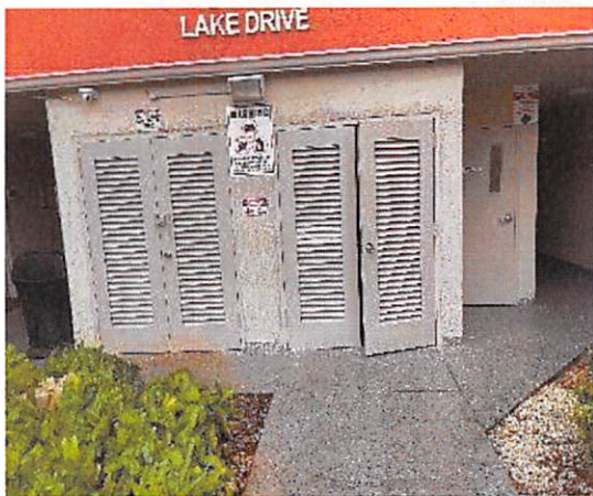
10.c Exterior doors in fair condition
