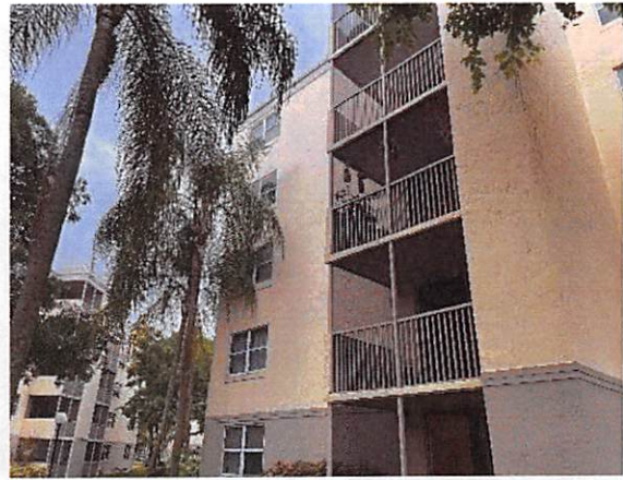
5.e Structure in fair condition
