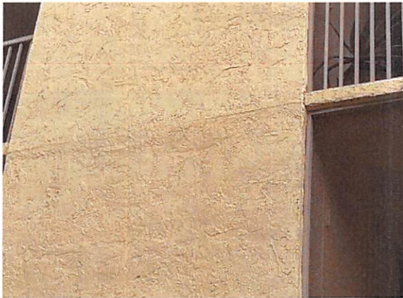
5.b Structure in fair conditions
