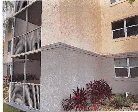
6.a Masonry wall in fair condition
