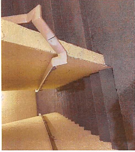
7.b.5 Guard rails in fair condition
